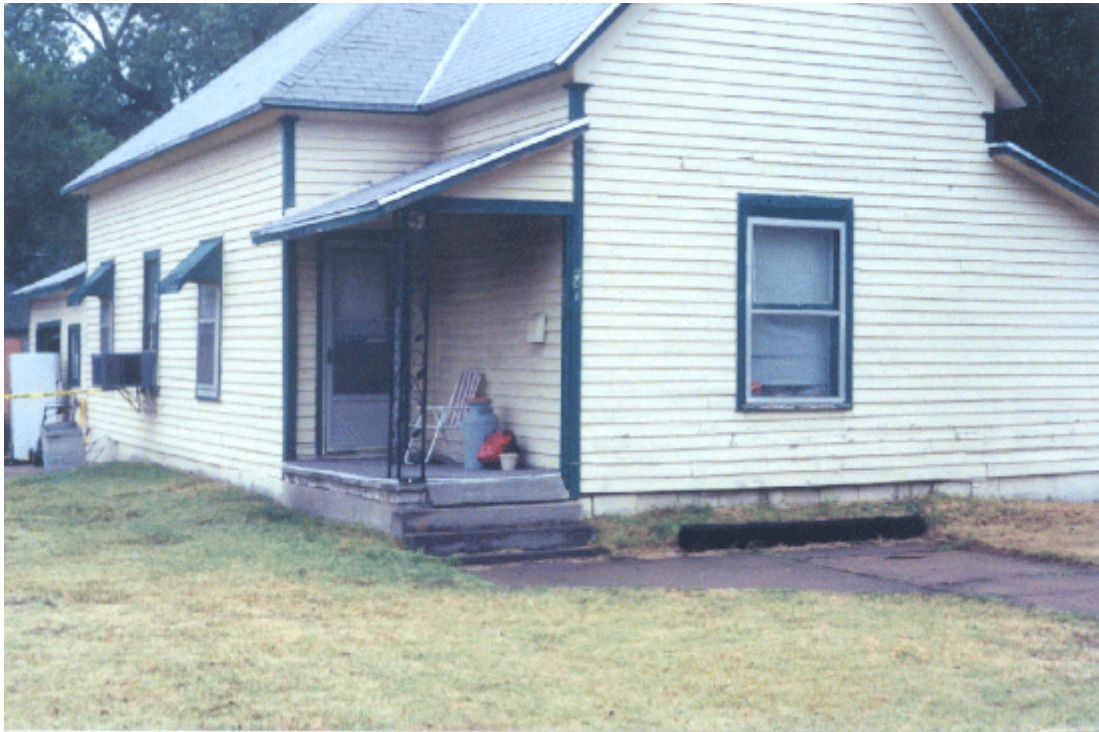
Windows and doors are closed, yet chemical odor detected.
